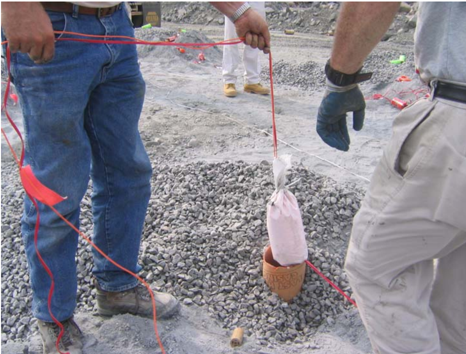
Figure 12 - Inserting top deck charge into blast hole
